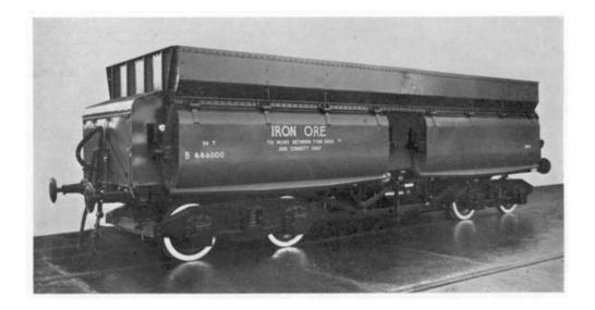
The Consett Ore wagon was built for the conveyance of iron Ore from Tyne Dock to Consett specially constructed wagons of 56 tons capacity have been provided. Each wagon is fitted with: -the: vacuum automatic brake and four power-operated side discharge doors which are under the control of the train locomotive driver.
